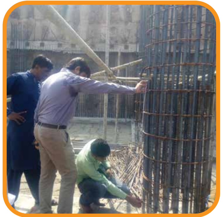
FIG#4 MEASUREMENT OF STEEL OVERLAP (MULTAN)
