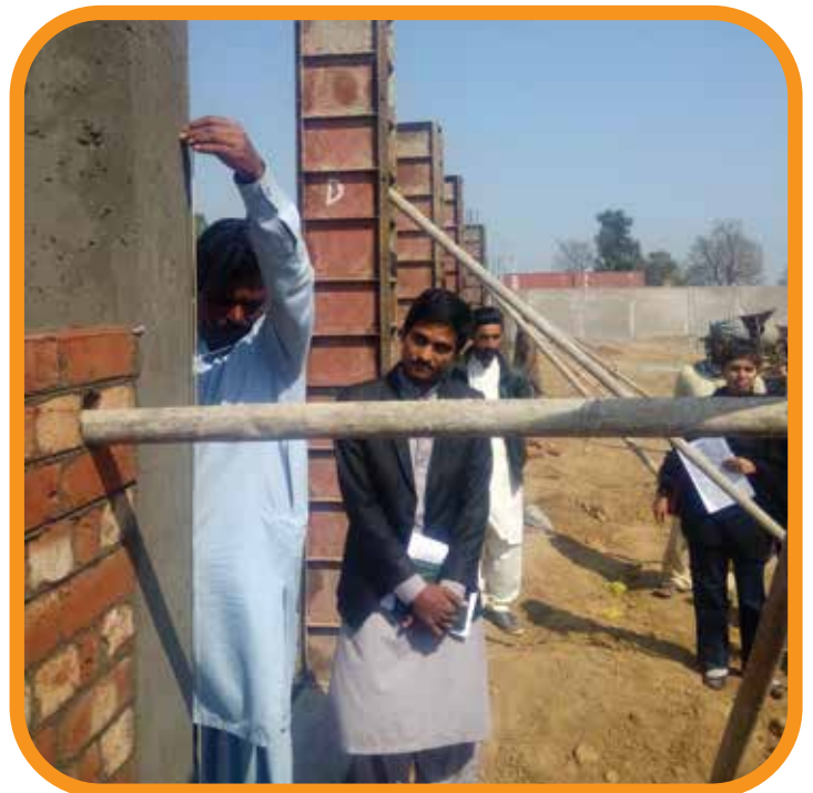
FIG#6 CHECKING OF VERTICAL COLUMN (JUDICIAL COMPLEX KAMONKI)
