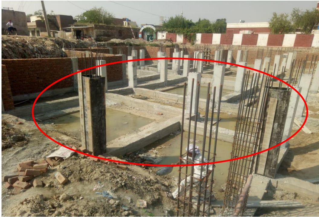
Figure No 7: Massive backfilling required
