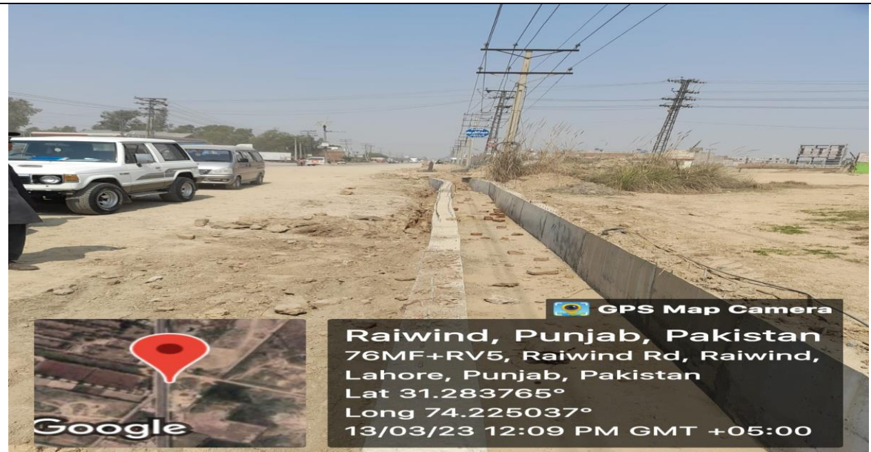
Fig No. 5: View of Side Drain
