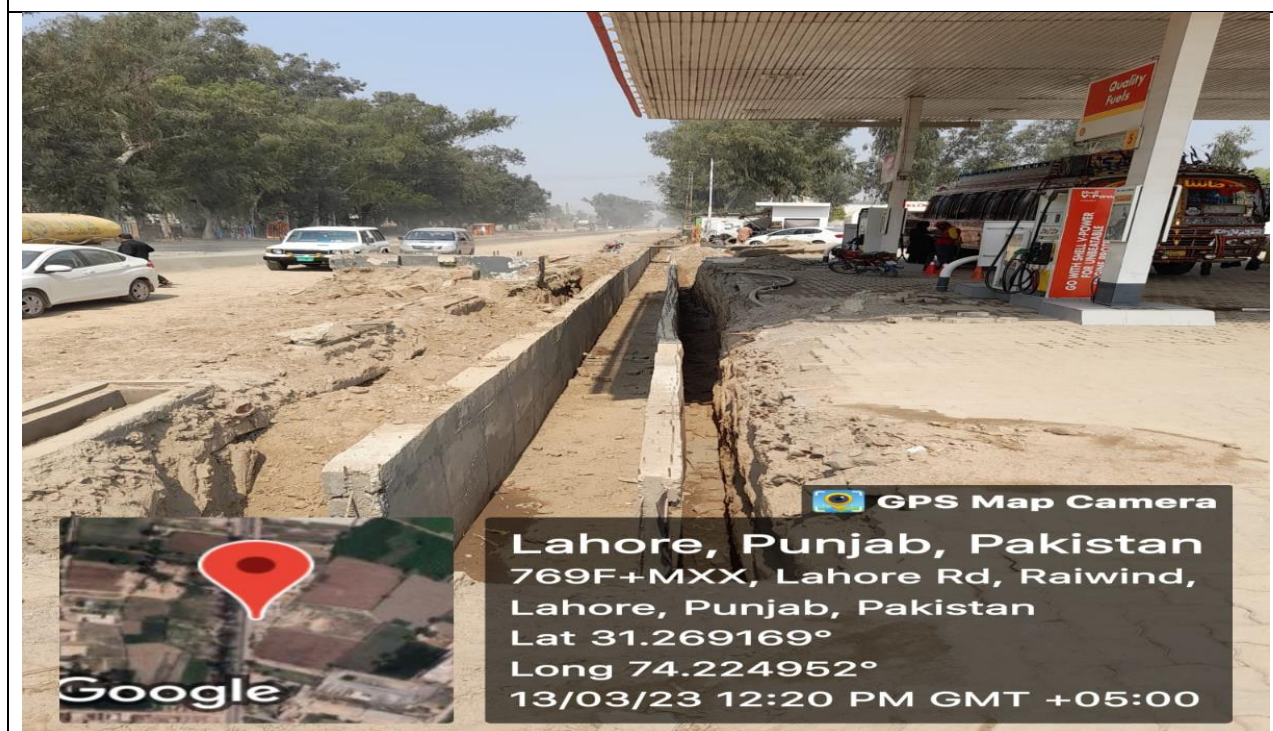
Fig No. 4: View of Side Drain
