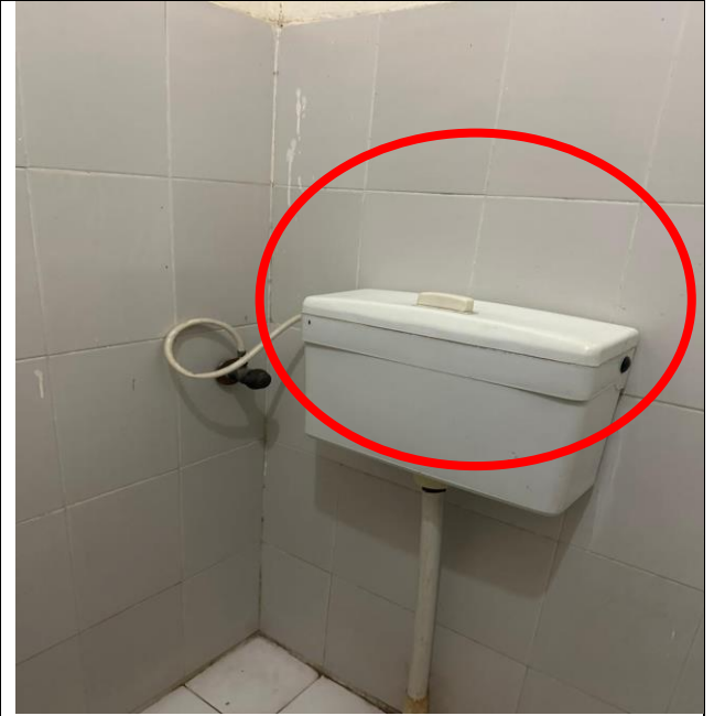
Figure 18: New cistern was installed
