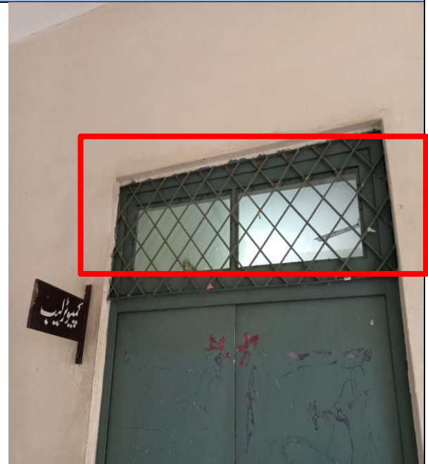
Figure 10: Glass of transom was reinstalled
