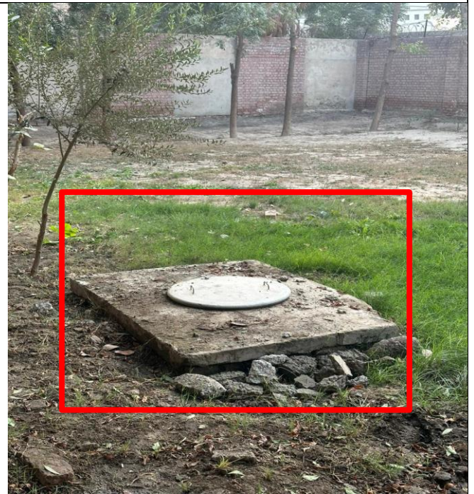
Figure 28: New man-hole cover was installed
