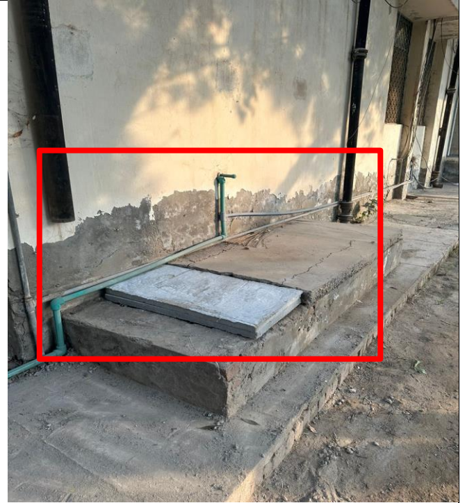
Figure 26: New slab of sanitary chamber was installed
