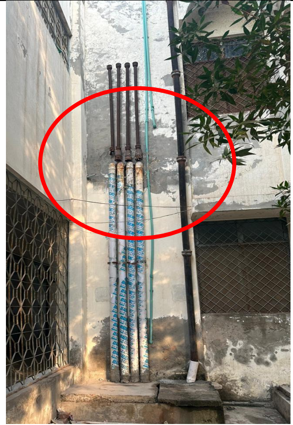
Figure 30: New sewer gas smell vent pipe was installed
